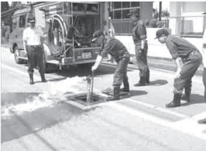
毎月定例の消火栓点検
