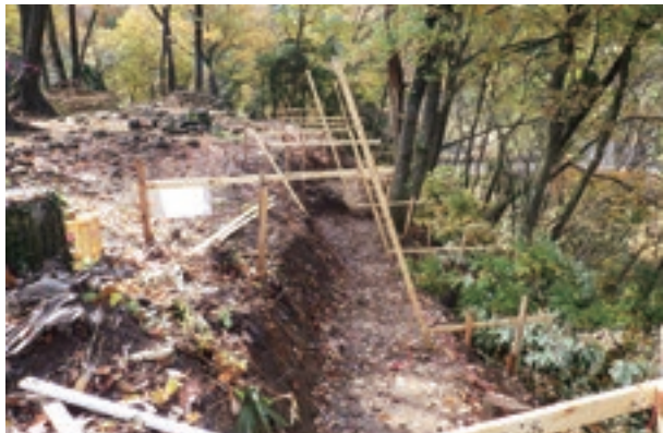
補強土壁工施工前
